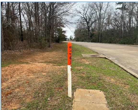
Fiber Optic in Neighborhood
